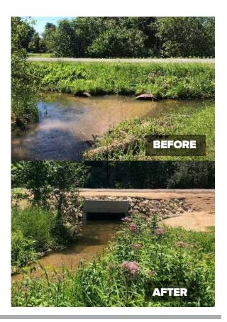
Several other 95-inch by 67-inch CSP arch culverts were replaced for private stream crossings, replacing 60-inch and 66-inch CSP culverts, which are necessary to meet the bank full width of the stream and improve flow conditions. From speaking with residents prior to bidding, we were able to eliminate several aging culverts that were no longer in use and were acting as obstructions in the Drain. In doing so, we were able to restore the natural stream in these locations.
