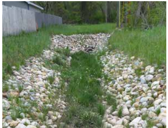
In-Line Detention areas constructed adjacent to existing residence
