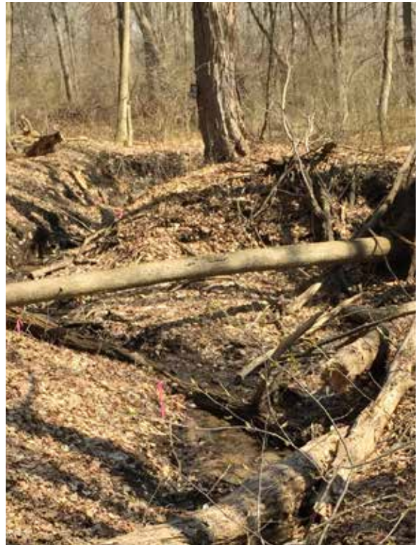
Downstream eroded ditch near North Shore Drive prior to construction
