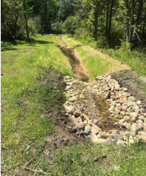
In-Line Detention area during construction
