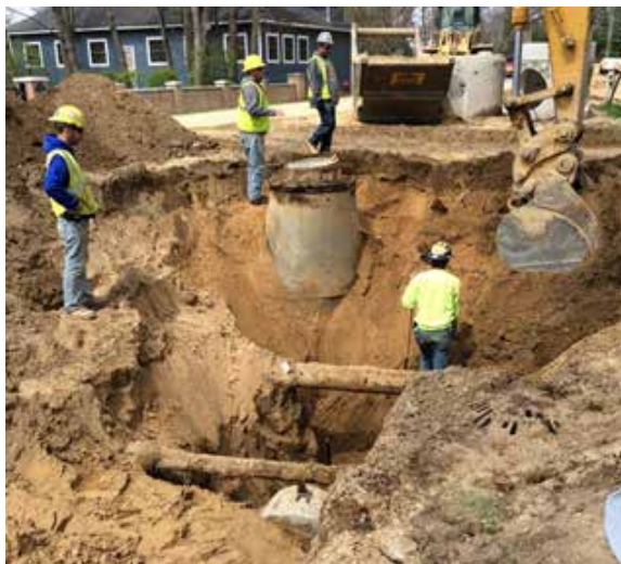
Working on utilities in the narrow right -of-way
