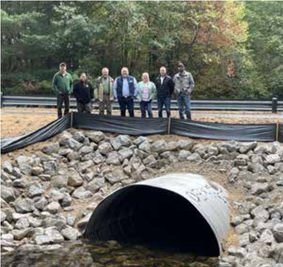
Project team at new culvert installation
