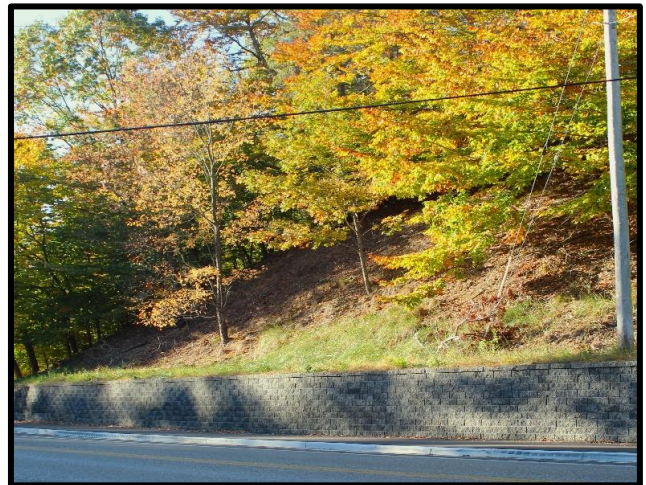
Retaining Wall at Lake Harbor and Hendrick After
