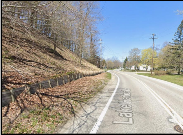
Retaining Wall at Lake Harbor and Hendrick Before
